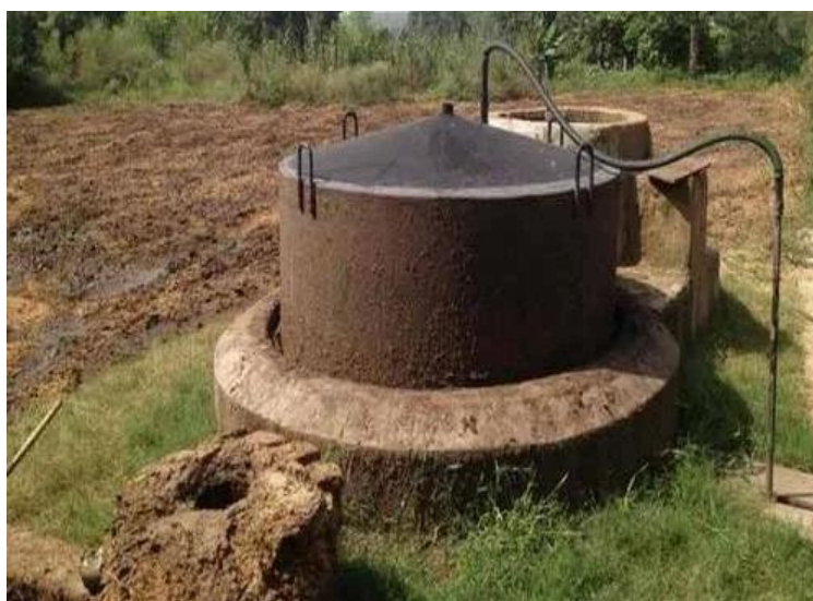
Picture3. Gobar gas plant provides clean energy and quality manure
